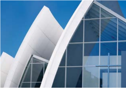
When used in building façades, Pilkington Optiwhite™ low-iron glass offers higher light transmission than conventional float glass.
