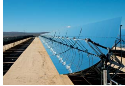
Concentrated solar power applications. Typically large area mirror arrays. Requires a large area and lots of sunshine. Particularly effective in sunny deserts.
