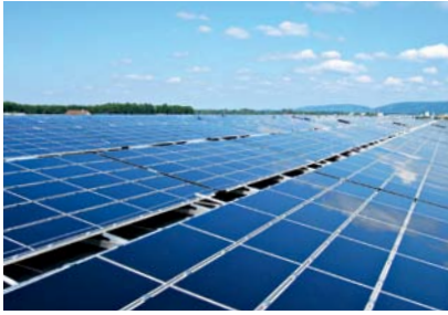
Thin film photovoltaic solar modules produce power at low cost per watt, but require large surface areas for installations.
