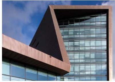
Increased focus is being placed on legislation and policies to improve the energy efficiency of buildings.
